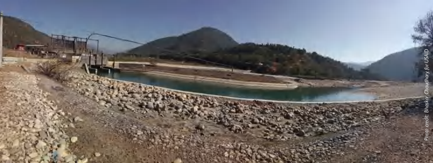
Jhimruk Hydropower dam in Jhimruk Watershed.
