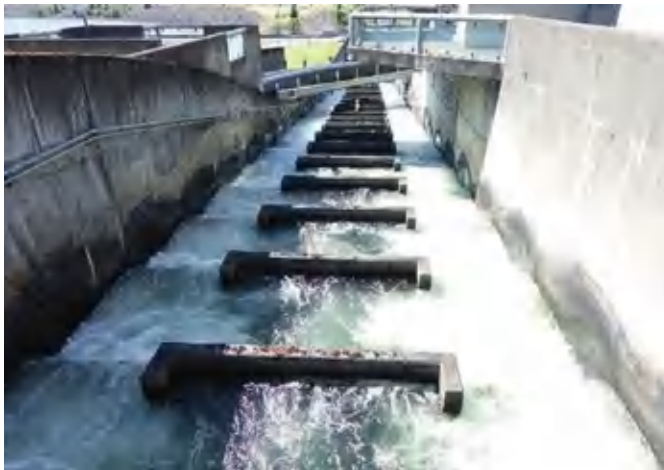
Fish ladder at Bonneville Dam
