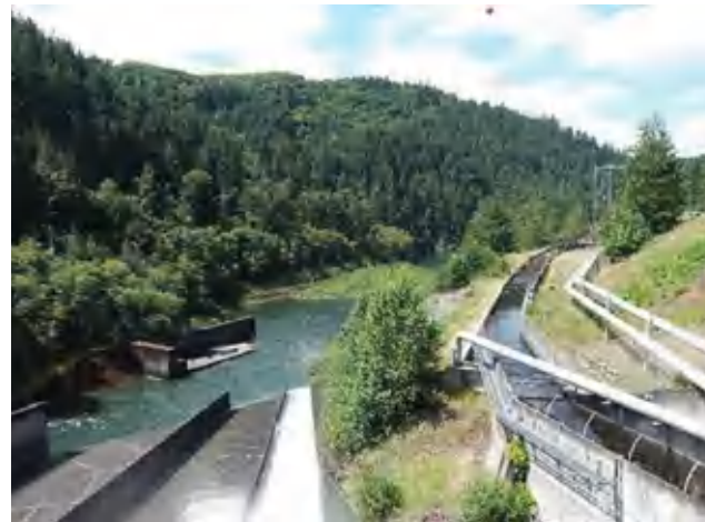
Almost 5km long fish ladder
